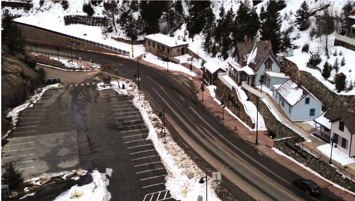
Black Hawk wants to give Central City $250,000 to annex the Briggs Lot (at left) into Black Hawk's city limits. The lot, which Black Hawk owns, adjoins High Street. It is across from the Gregory Point Victorian historic homes and a dozen yards uphill from the west end of Gregory Plaza.
